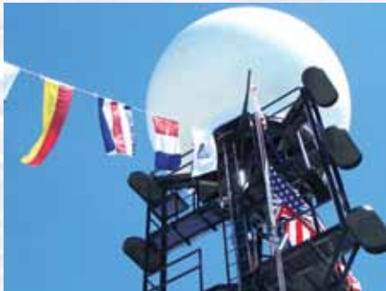
Okeanos Explorer 's prominent VSAT (Very small aperture terminal) dome enables satellite communications between explorers ashore and at sea and provides multiple high-definition video streams for widespread dissemination. Image credit: NOAA.
