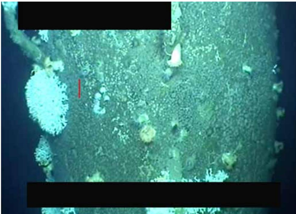
**Figure 12.** *Lophelia* coral #5 growing on Rig Platform C. Structure Diameter = 320 cm. Image made 17 years after structure was placed in the water. Image courtesy Chuck Fisher Lab, Penn State University.
