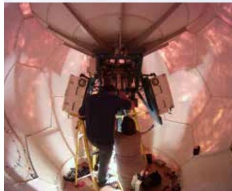
Technicians work to repair the satellite antenna in the VSAT dome. Image courtesy of NOAA *Okeanos Explorer* Program.
